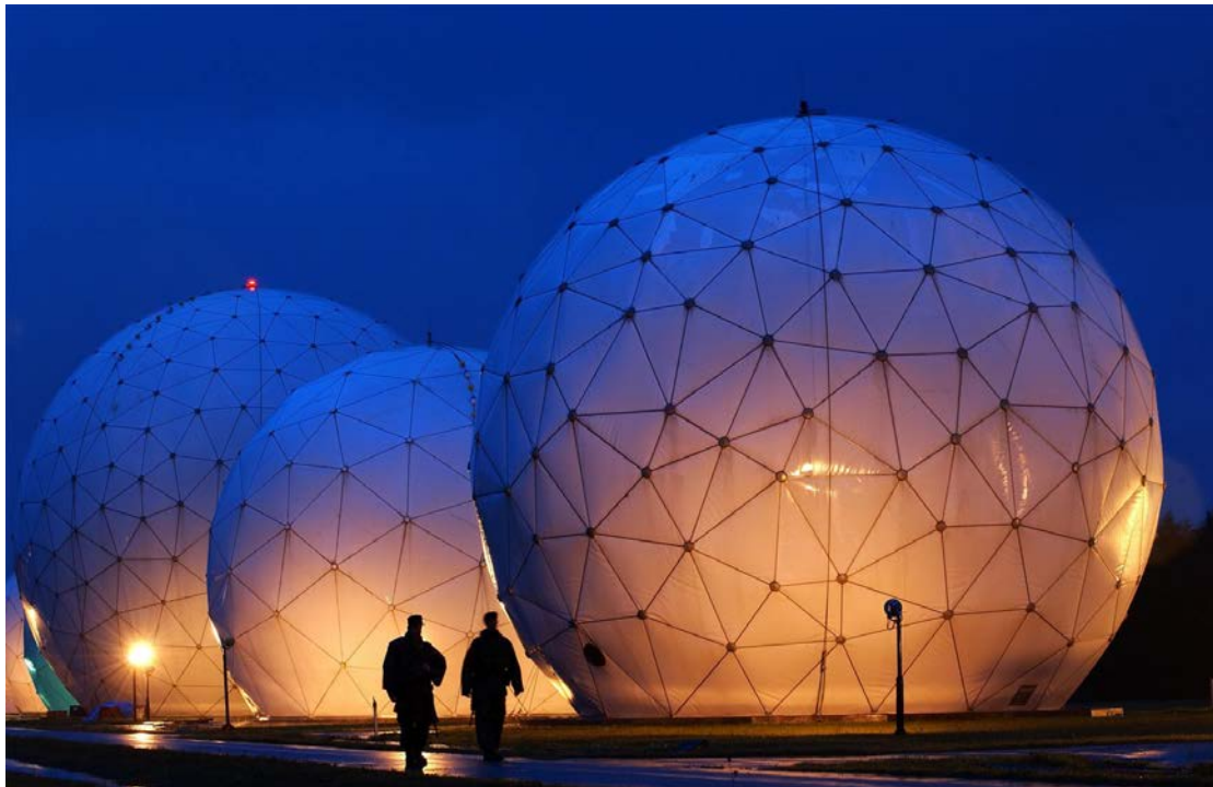
'Radomes' at the encryption operations centre, Misawa airbase, Japan. The portmanteau word 'radome' is derived from 'radar' and 'dome' and describes a weatherproof enclosure that protects an antenna. © Preston Keres - Source: www.kereskreatives.com .
