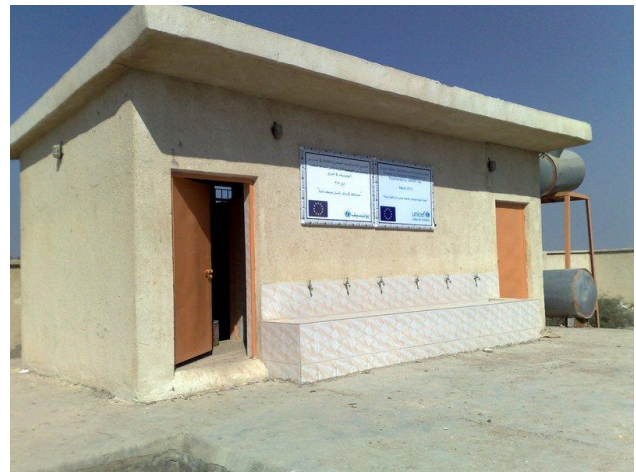
A rehabilitated latrine and hand washing facility in Al-Khahla'a school, Missan as part of an EU funded project implemented by UNICEF (Photo: UNICEF)
