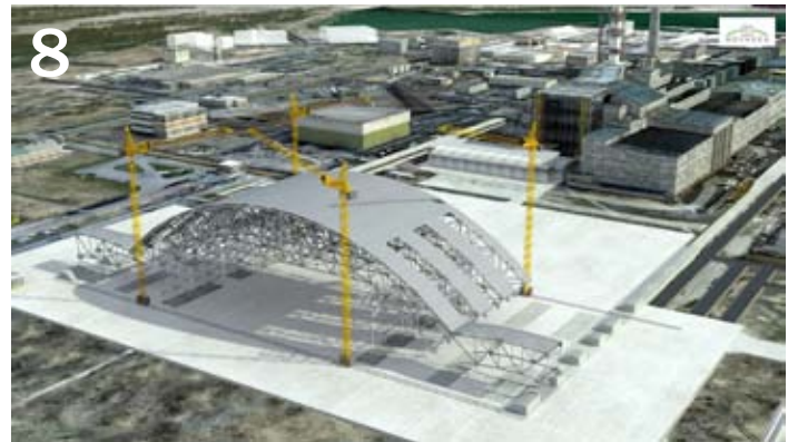
Shelter segments lifted and further elements added to create first section
