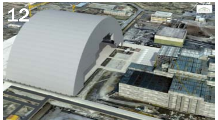
Whole structure slid into place over object shelter
