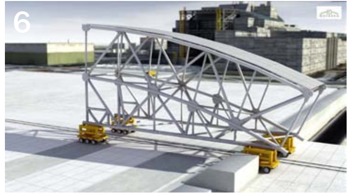
Prefabricated NSC elements transported to site
