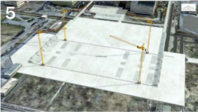
Lifting cranes and sliding pad elements installed
