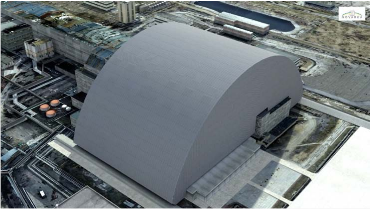
Final structure will cover unit 4 and object shelter for at least 100 years
