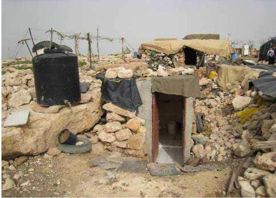
Susya toilet under demolition order by the Israeli army © AI
