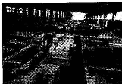
Building of the anode plant
