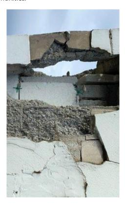
However, a study carried out by Leemann et al using in-depth microstructural analysis found that the damage in the homes is likely due to internal sulfate attack, particularly triggered by pyrrhotite oxidation. The authors suggest that the presence of mica in concrete blocks can affect compressive strength, but that
