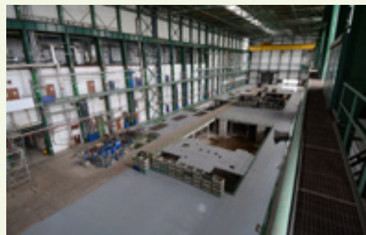
2015: Turbine hall without turbines © Javys.
